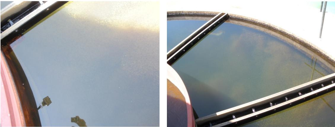
The sedimentation/flocculation was improved and aluminum sulphate needs were reduced providing savings of around 30 Euros per day as well circa 50 Euros savings in sodium hypochlorite. During winter and better water quality more savings are expected.
