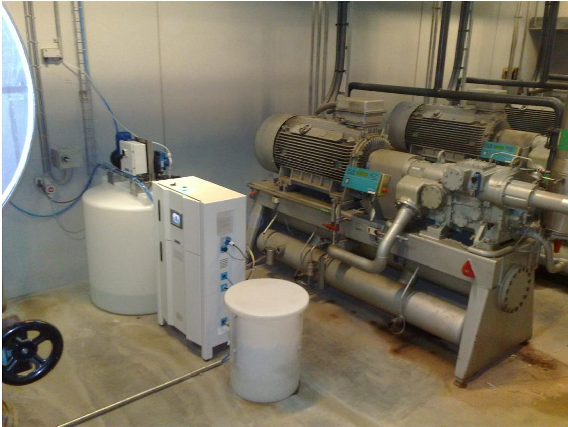
An ORP sensor was installed in the system and connected to a dosing pump. The set point for the ORP (Oxygen reduction potential) sensor was 550mv. At this level there should be no significant bacteria levels present. The pump starts and doses into the system when the ORP starts to drop below this level maintaining a continuous hygienic environment for the product.
